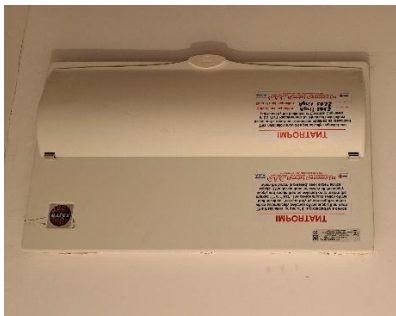
Fig. 1 Consumer Unit Exterior
